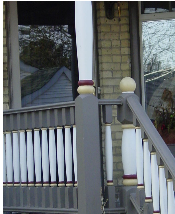
Well restored porch with new millwork at 850 Lorne
