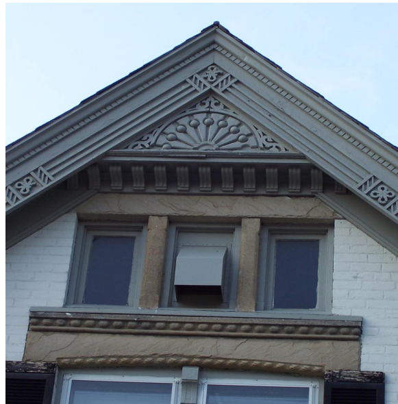
Decorative stone trim on windows
