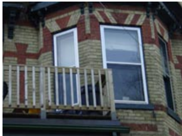
Multi-coloured brick masonry details
