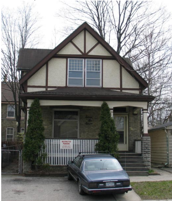
Example of original stucco finish that appears on a number of homes in Old East
