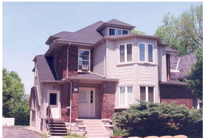
Substantial alterations were undertaken to the exterior facade of the original dwelling, with respect to removal of original features, additional doors, etc. Where possible, such alterations should be minimized.
