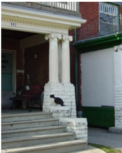
Pre-cast concrete porch columns and piers
