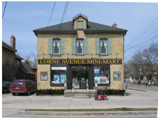
New lighting, poster boards, newel posts & planting.
