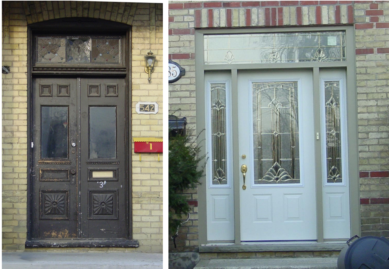
Examples of original doors (left) and replacement doors (right) in Old East
