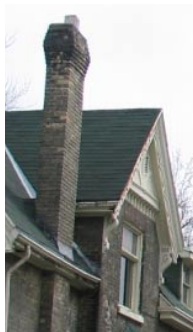
Decorative masonry details in chimney
