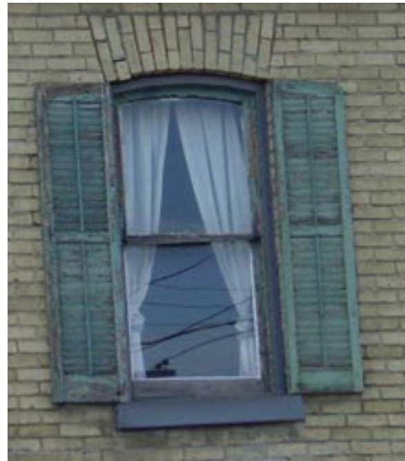
Example of original louvered wood shutter that conforms to window opening. Shutter exhibits some effects of exposure to weather.
