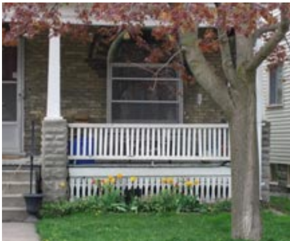
Porch with pre-cast concrete pier, wooden column, railings and balusters, decorative skirt
