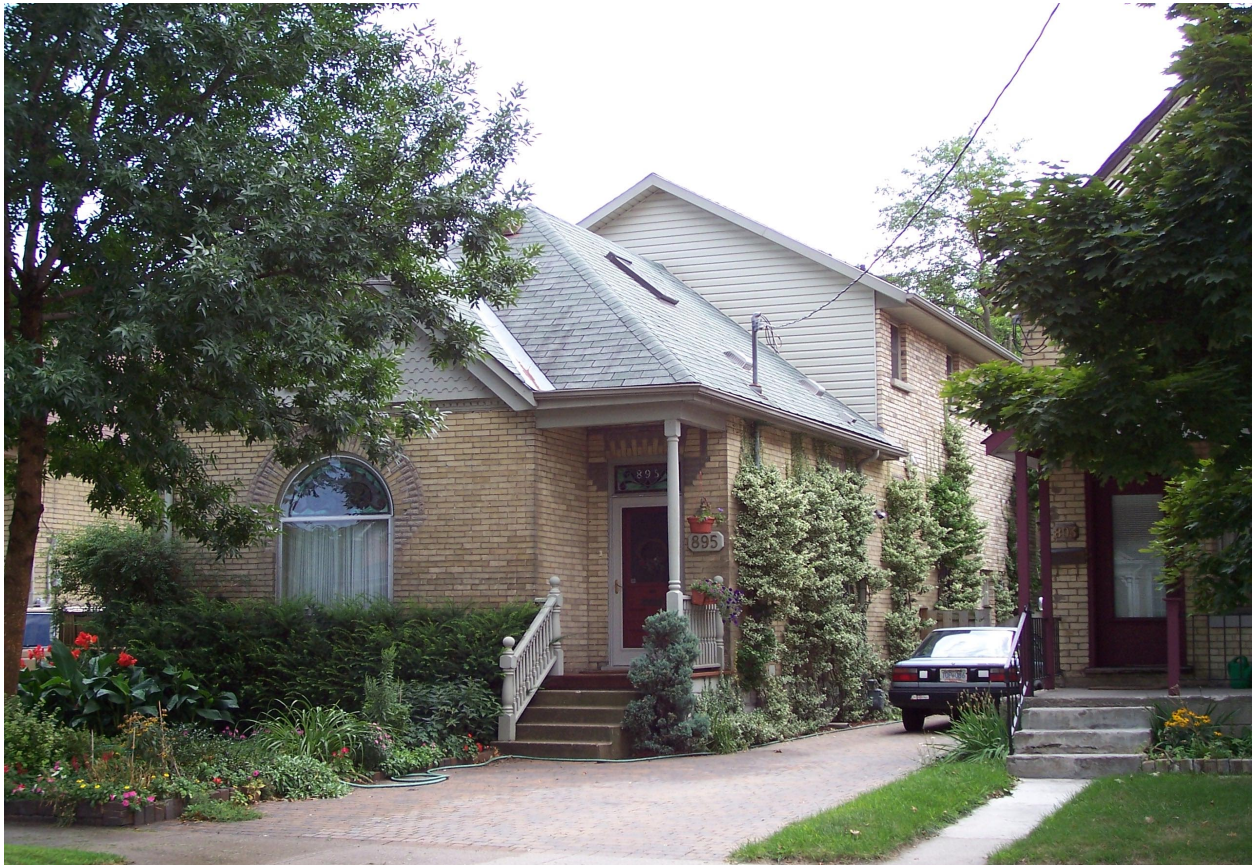
New addition is distinguishable from the original dwelling and illustrates good sensitivity to original dwelling through slope of roof, height, use of colour and materials
