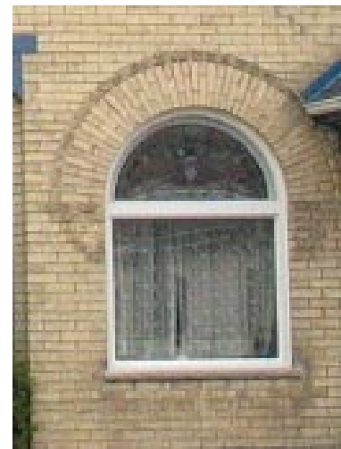
Typical arched window found in many Old East dwellings
