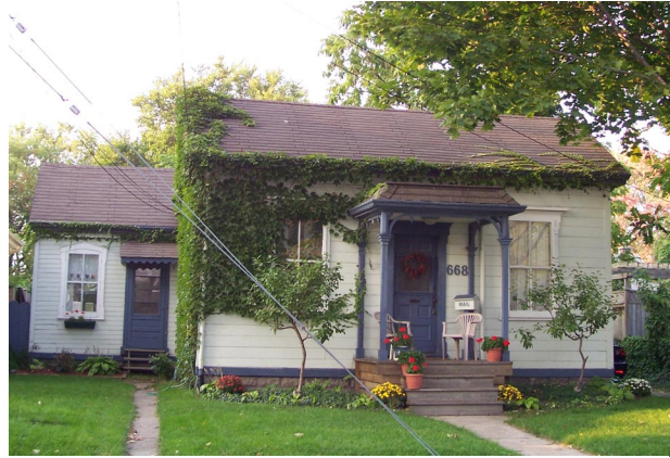
Traditional use of wood siding and trim
