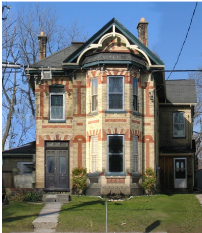
Remove existing porch
