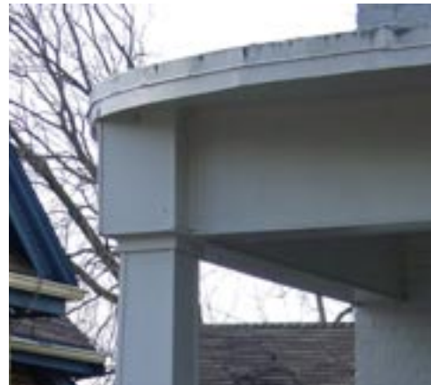
Avoid re-cladding soffits and fascias with metal or vinyl materials
