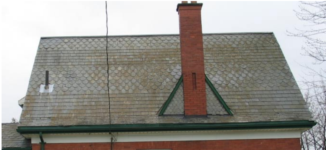
Decorative slate patterns in roof
