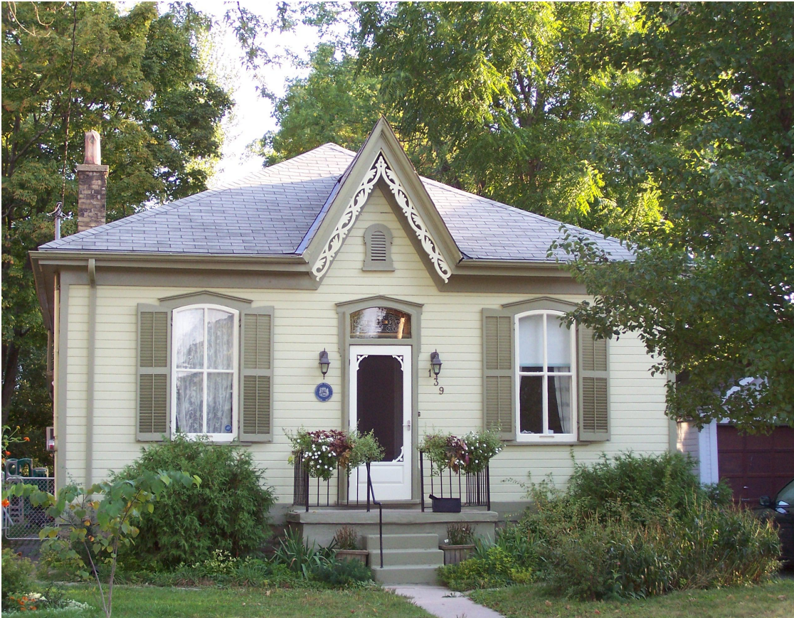
Example of retained and well maintained original shutters. Example also illustrates preferred types of storm doors and storm windows (wooden) for typical doors and windows in Old East.
